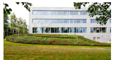
Office buildings West-End - Brussels Periphery (BE)
