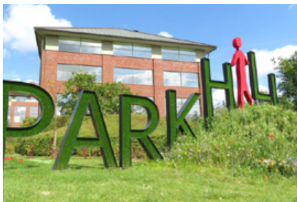
Office buildings Park Hill - Brussels Periphery (BE)
