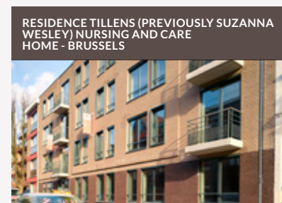
RESIDENCE TILLENS (PREVIOUSLY SUZANNA WESLEY) NURSING AND CARE HOME - BRUSSELS Surface area: 4,960 m 2 Number of beds: 87 Lease: 27 years - "triple net"
