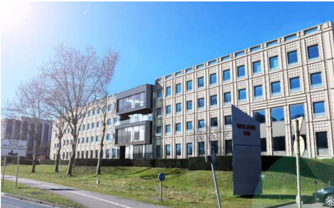
Woluwe 106-108 nursing and care home - Brussels (BE) (projected situation after completion of work)
