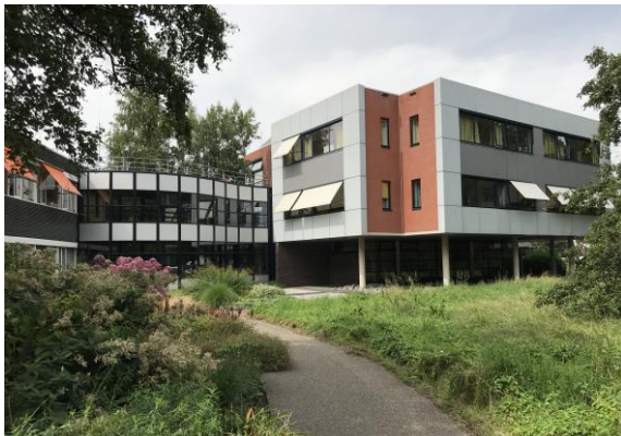
Actual situation before works
