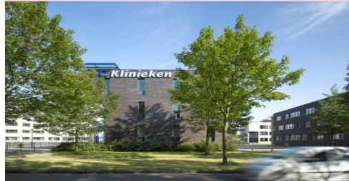
Medical care centre - 2,380 m 2 Almere - DC Group
