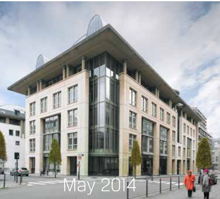
Letting of the Brussels office building Livingstone II for 15 years to the European Commission
