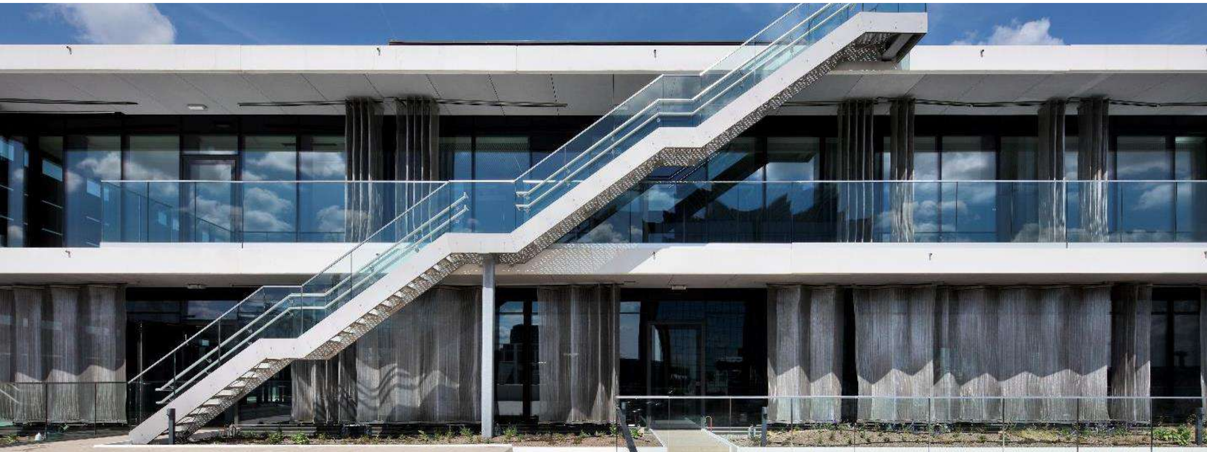
Quartz Office building – Brussels CBD
