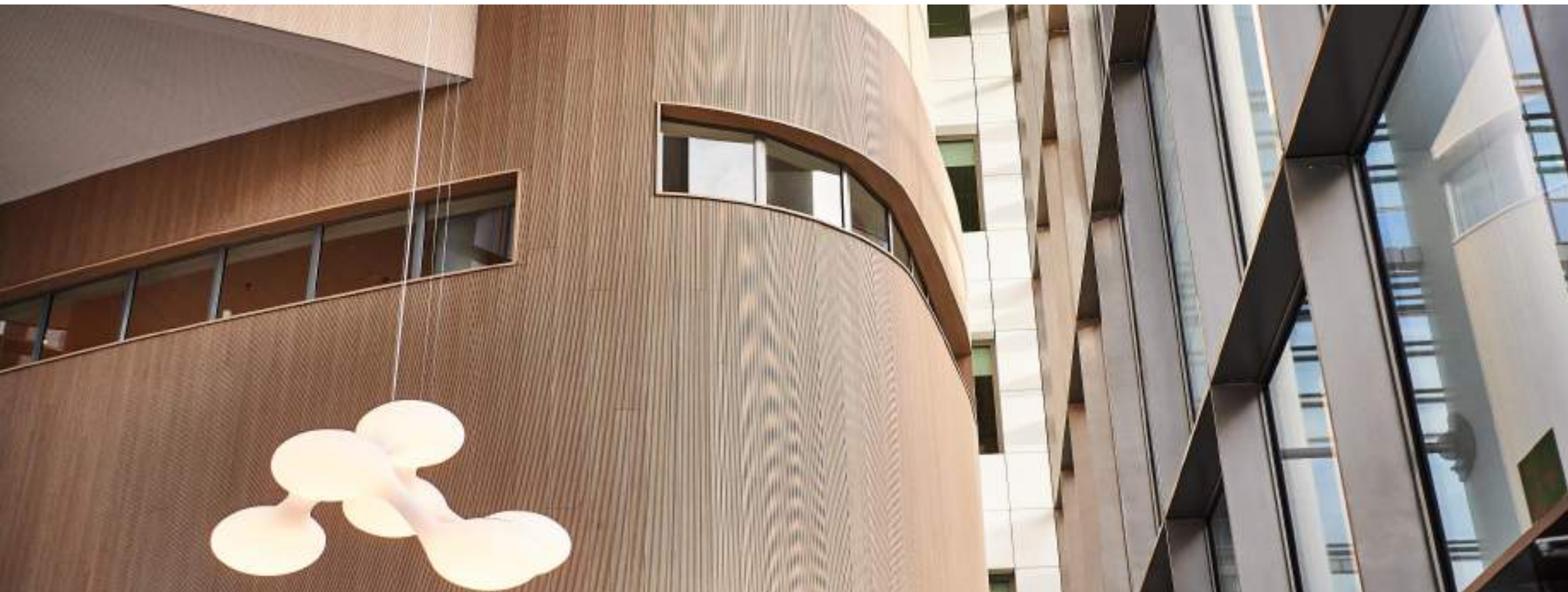
Belliard 40 office building - Brussels CBD
