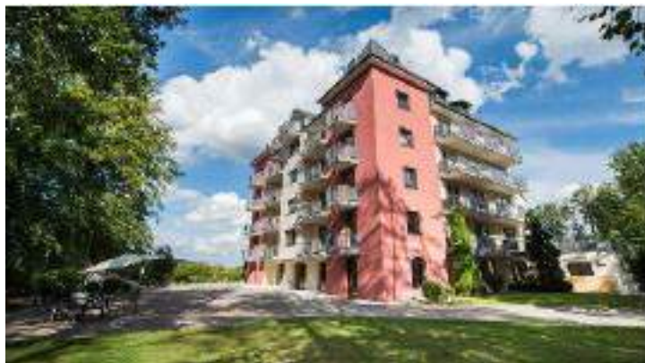
Nursing and care home Parkhöhe – Lindenfels
