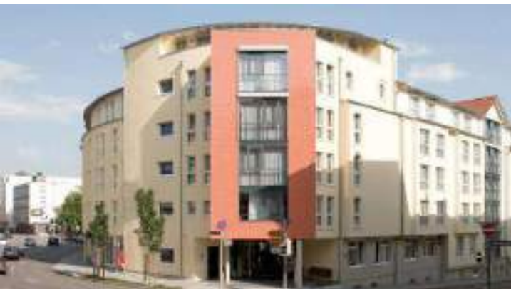
Nursing and care home Haus Osterfeld – Pforzheim
