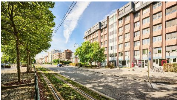
Office building Souverain/Vorst 280 - Brussels
