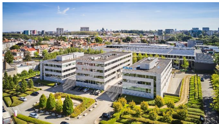
West-End Office Park – Noordkustlaan 16 A-B-C – Grand-Bigard
