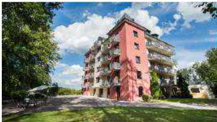
Nursing and care home Parkhöhe – Lindenfels
