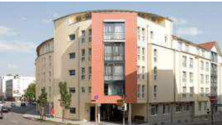
Nursing and care home Haus Osterfeld – Pforzheim
